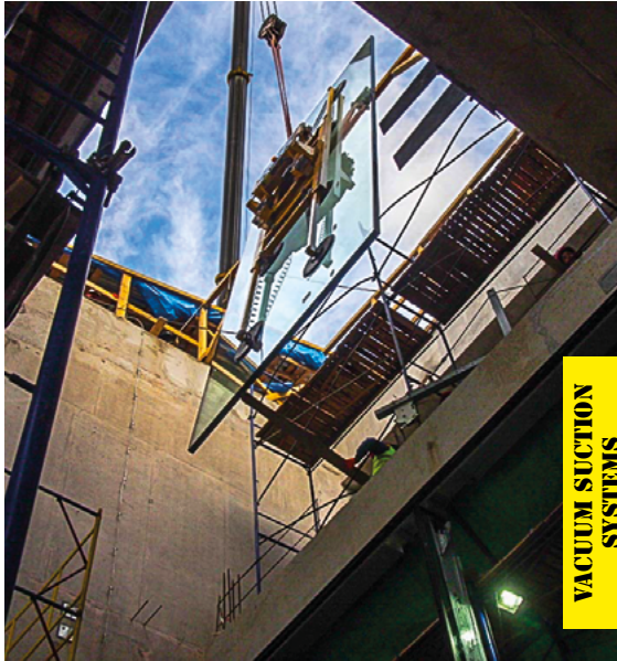
Mounting of 9x3 m-pane SNEGIRI-ECO in Moscow at -10°C
