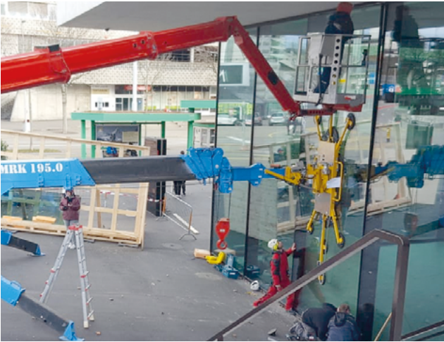
Manipulator VSGU1600K and assembly crane MRK 195 in action: 1.2 t pane, glazing under protrusion (St. Jakobshalle in Basel, Switzerland)
