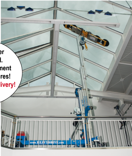
ML79 assembly lift and overhead vacuum suction system in a narrow space
