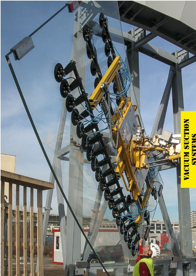
Victoriei Office Building in Bucharest / Romania Placing a spherically curved pane, H 4,783 x W 2,762 mm
