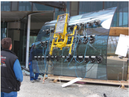
Fig. above: Rund 4 Wien, Vienna; Placing 500 kg curved panes
