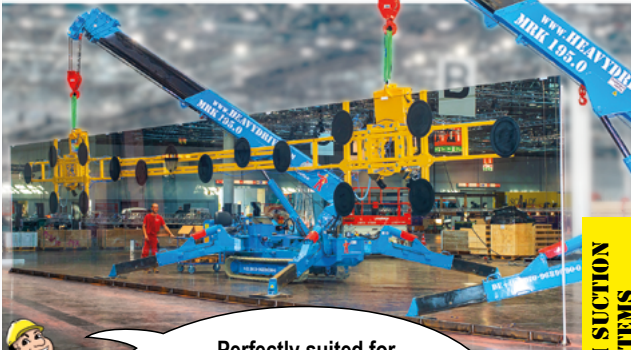
Glasstec 2018: Mounting of world record pane measuring 18 m long, 3.2 m tall and 4 tonnes in weight
