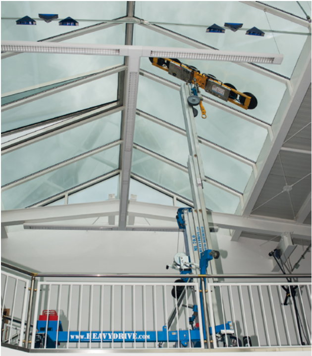
Image above: Assembly lift ML79 and Overhead vacuum suction system working in tight space Image below: BV Miami Aventura Mall, USA
